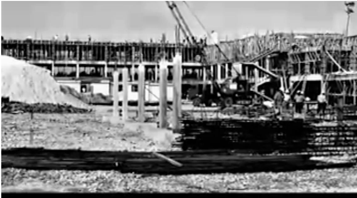
Jansel Court building in construction 1968
